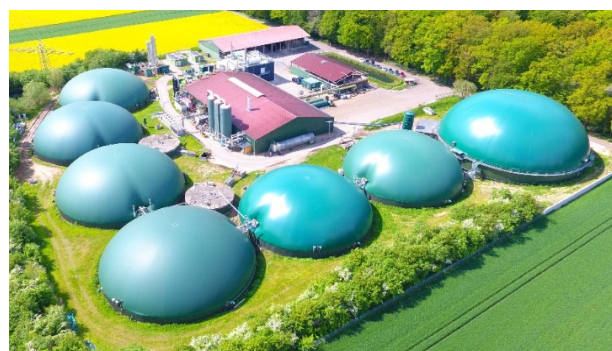
Figure 1. Aerial photo of the demonstration plant BENAS.
