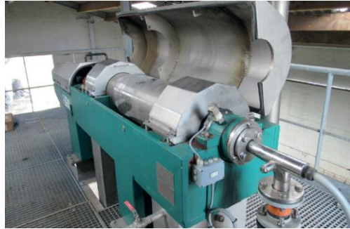
Figure 2-1 Horizontal decanter centrifuge Source: (Gorissen and Snauwaert 2018)
