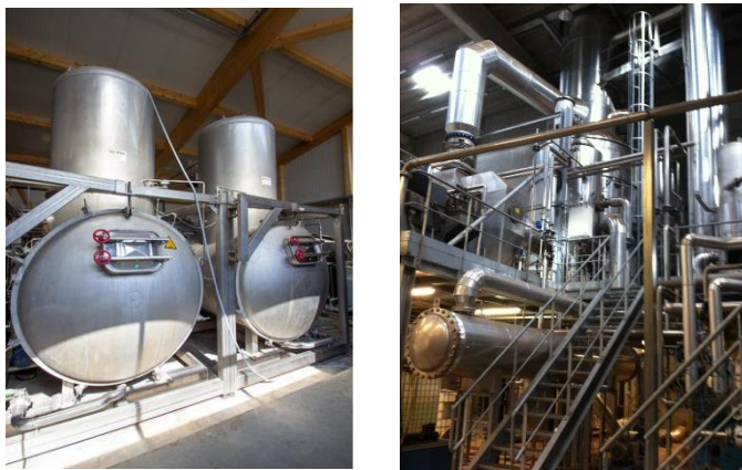
Figure 2-20 Evaporators in different configurations and sizes. Source: (Kühne 2018)(left), Waterleau New Energy
