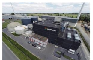
Waterleau BV, a mesophilic anaerobic digestion plant in Ypres (80 km west of Ghent), West-Flanders, Belgium, in operation since 2012 with a total annual substrate treatment capacity of 120,000 tonnes. Processing manure and biowaste.
