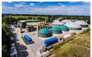
**Groot Zevert Vergisting B.V.**, a mesophilic anaerobic digester plant in Beltrum (35 km southwest of Enschede), Achterhoek Region, Province Gelderland, The Netherlands, in operation since 2004 with a total annual substrate treatment capacity of 135,000 tonnes. Processing pig manure and residues from agro-food industry.
