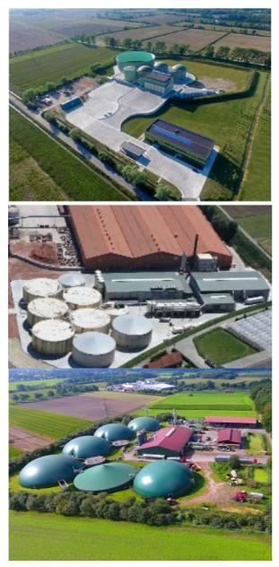
Acqua & Sole S.r.I., a thermophilic anaerobic digestion plant in Vellezzo Bellini (30 km south of Milan), Pavia, Lombardy, Italy, in operation since 2016 with a total annual substrate processing capacity of 120,000 tonnes. Processing municipal sewage sludge and source separated domestic food waste.
