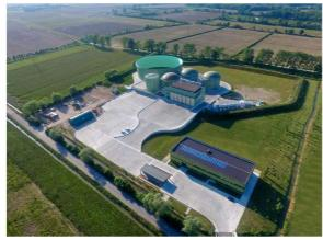
**Acqua e Sole S.r.I.**, a thermophilic anaerobic digestion plant in Vellezzo Bellini (30 km south of Milan), Pavia, Lombardy, Italy, in operation since 2016 with a total annual substrate processing capacity of 85,000 t. Processing municipal sewage sludge and source separated domestic food waste.
