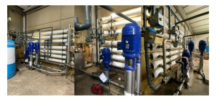
*Figure 2.3 The new reverse osmosis unit installed at the demonstration plant AM-Power (2020).*
