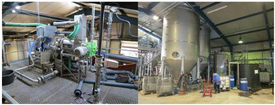
Figure 1.1 Photos of the new RePeat installation at Groot Zevert Vergisting (left; screw presses, right; stainless steel settling tank, stainless steel precipitation tank and a black buffer tank).
