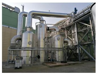
Figure 3.2 Photo of the N absorber installed at the demonstration plant <u>Acqua&Sole</u> (2020).
