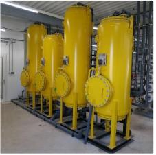
Figure 1.2 Photos of the GENIUS installation for the production of solid fraction of digestate, NK concentrate and clean water from digestate.
