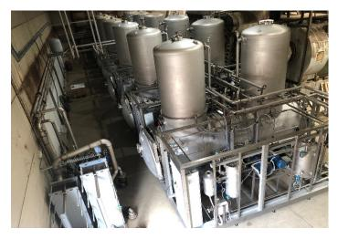
Figure 2.1. The new evaporator units installed at AM-Power.
