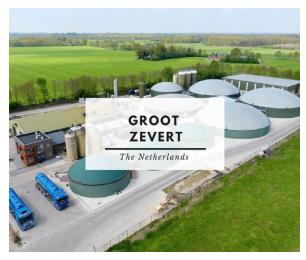
**Groot Zevert Vergisting B.V.** was set up in 2004 in response to the surplus of manure in the region and the profitable conditions for biogas production. It now processes, through mesophilic digestion, over 100kt tonnes per annum of pig manure and agro-industrial organic waste. This year, the plant will be extended with a novel nutrient recovery installation converting the digestate into valuable mineral fertilizers and organic soil improvers.
