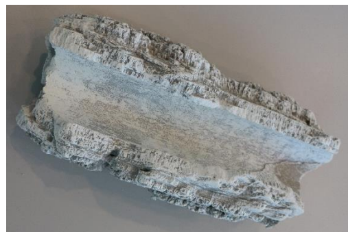
Figure 1. Struvite depositions in the pipes to the sludge holding tank
