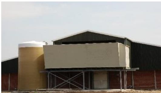
Photo 1: air scrubber (left) and ammonia stripping / scrubbing installation (right) (© VCM)
